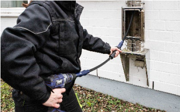
Fig. 3: Using the push rod with handle (article 11270)
