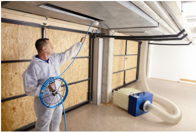
Fig. 33: Cleaning ductwork with a roller guide ball and compressed air whip, dirt extracted with dust collector
